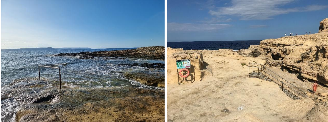
Figure 2.5. Handrail installed on the entrance of Ras il-Hobz dive site (left) and steps for safer descent to shore and entry point at Dwejra (Blue Hole) dive site (right).
