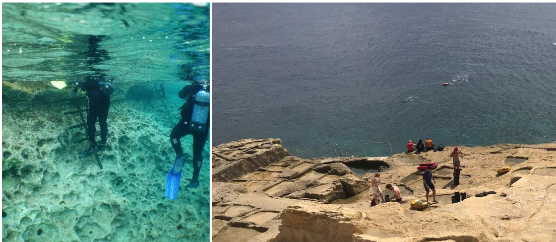
Figure 2.6. Ladder installed at Xatt I-Ahmar dive site as seen from in water and above.
