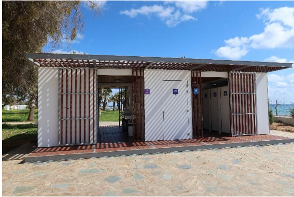
Figure A44. Bathrooms and changing facilities.
